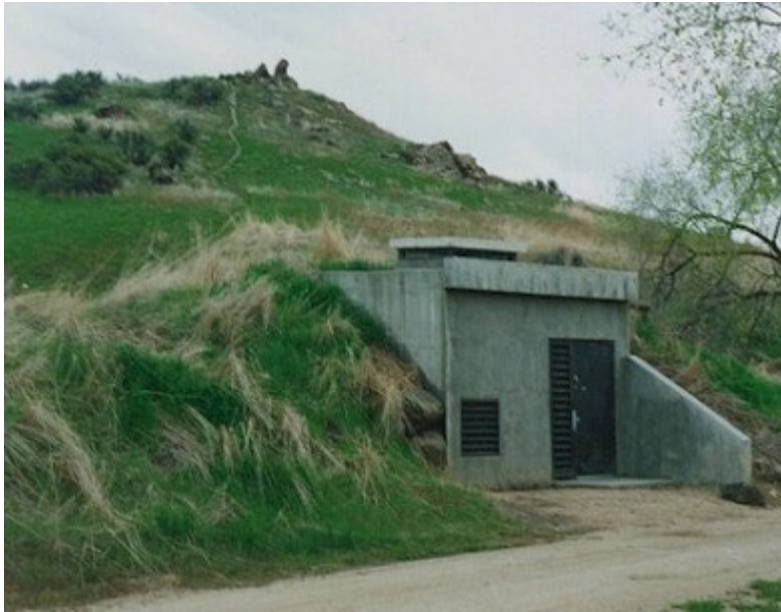
Figure 6 - Wellhouse for one of the City of Boise's geothermal production wells.
