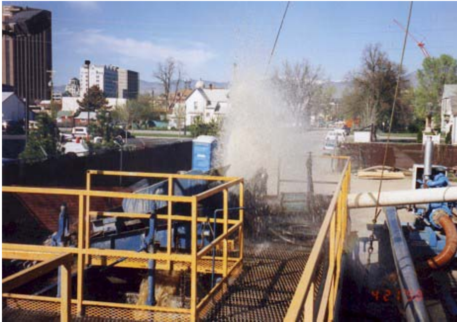
Figure 8 - In 1998, the City of Boise drilled a well to re-inject spent geothermal fluids into the aquifer.
