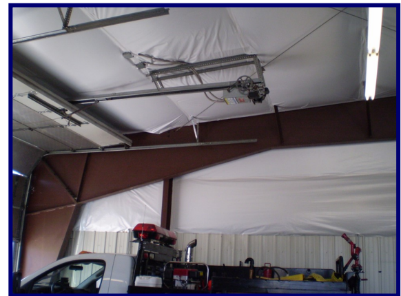
Lava Hot Springs Fire Station Insulation Project
