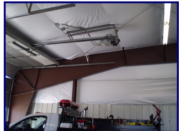
Lava Hot Springs Fire Station Insulation Project
