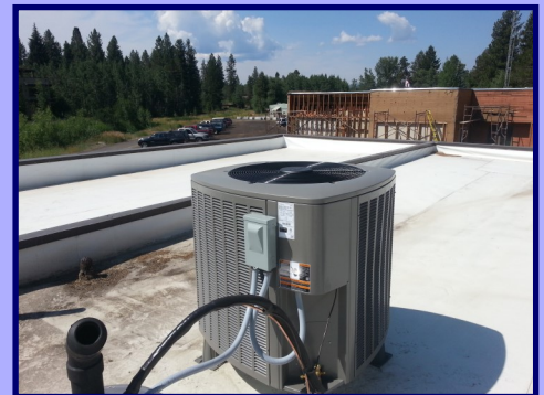
McCall Library Furnace Replacement Project
