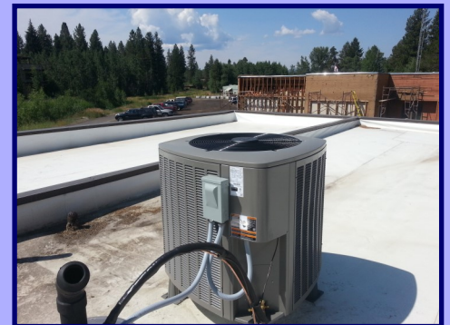
McCall Library Furnace Replacement Project
