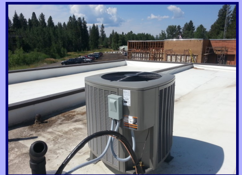
McCall Library Furnace Replacement Project
