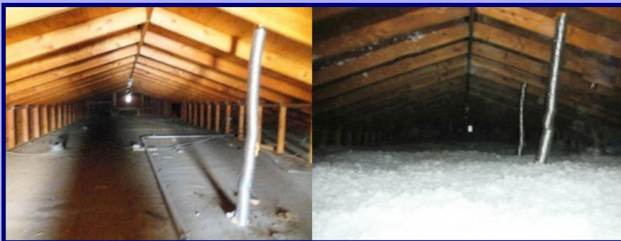
Cassia County Assessor's Office Attic Air Sealing & Insulation Project
