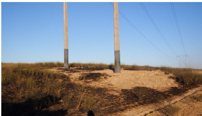
Figure 20: Vegetation management and fire-resistant mesh wrapping on Idaho Power transmission poles. This project was funded, in part, through the State of Idaho's Energy Resilience Grant Program.
